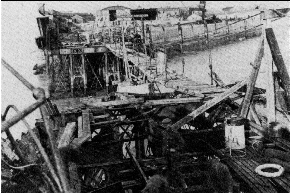
The gap torn in the Zeebrugge Mole viaduct by the British submarine. This photograph, taken just after the war, shows the temporary structure in place to bridge the gap.
